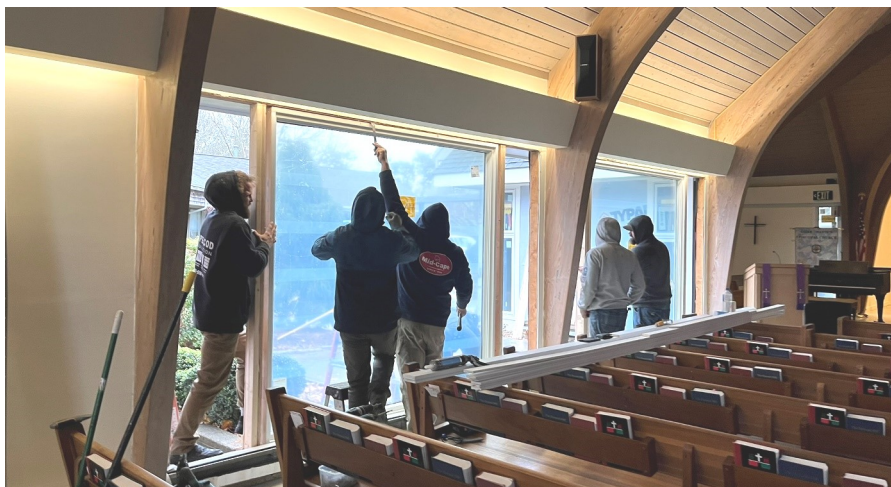
New windows being installed in the Sanctuary.
